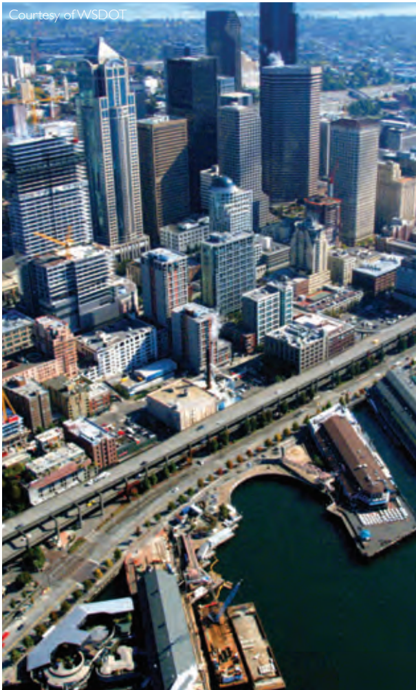
Seattle shoreline before demolition of the viaduct
