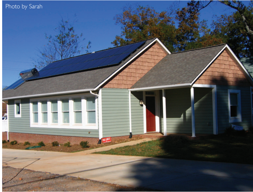
Zero Energy House in the Ridgeview Neighborhood of Hickory, N.C.
