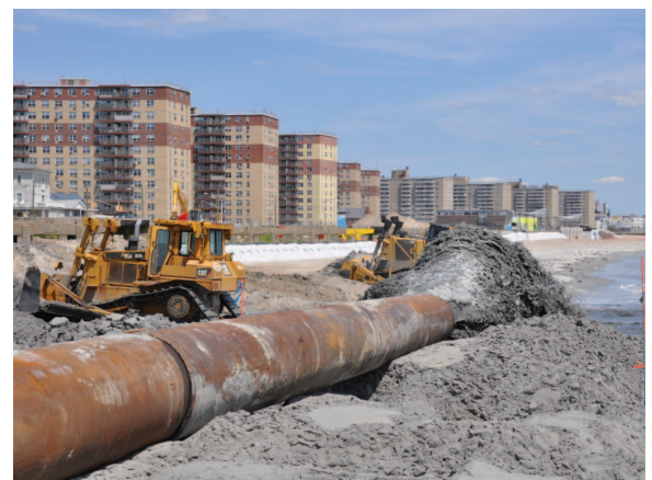
Post-Sandy sand placement at Rockaway Beach. Approximately 3.5 million cubic yards of sand is placed to reduce risk from future storms.
