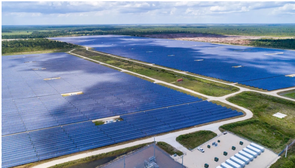
The Babcock Ranch Solar Farm
