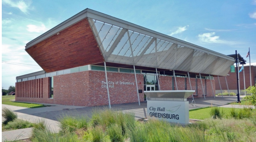
Greensburg City Hall
